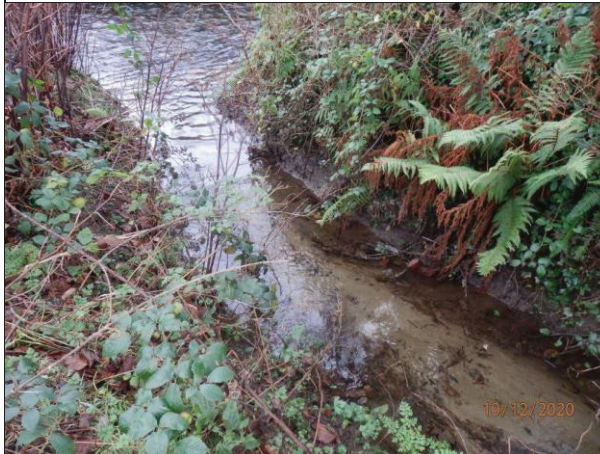
View d/s to the confluence of with the Burnfoot River. Note the extensive coverage of sand and silt on the riverbed.
